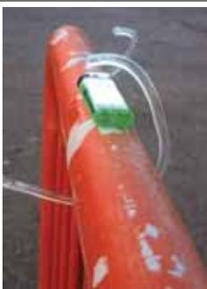
*January 2007. This photograph shows an icicle on the railing outside the Annagh Medical Centre, Doctor's Road, in January 2007. What appears to have happened is that water inside the railing froze, expanded and was pushed outwards through a small circular hole in the metal. As it did, the colder temperature outside froze it further it kept expanding, causing the icicle, which eventually curved nearly all the way around the railing! Cigarette lighter shown for scale.*
