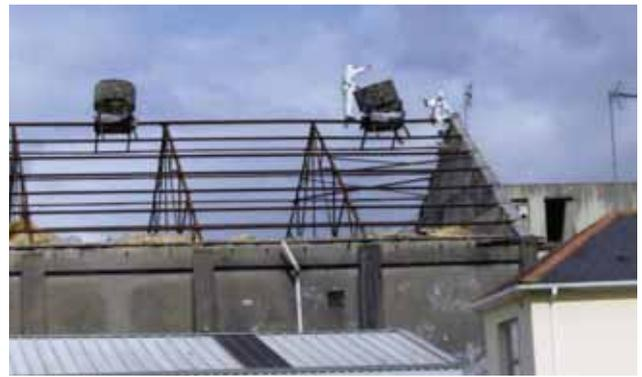
*These images were taken in the spring of 2008 when workmen attached to harnesses and wearing protective masks and white body suits began dismantling the old asbestos roof. It took many weeks to complete this part of the project. The first image was taken on 27th March and the second image was taken on 8th April.*
