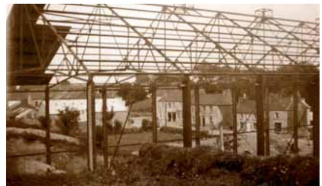
*Steelwork of the Star Cinema being erected in 1945, with houses in Clare Street visible in the background.*
