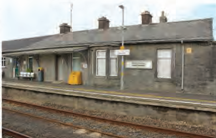
Ballyhaunis Station, opened in 1861, built with limestone block walls and with a canopy supported by four large, very ornate cast iron brackets. There is a modern extension at the Westport end (now the booking office). The bay window and the window to the right are in the former Station Master's residence.
