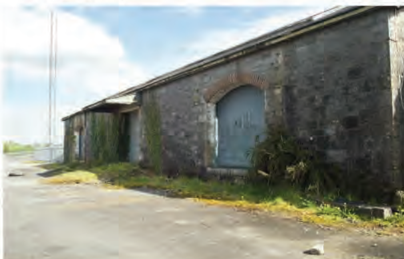
The goods sheds.
