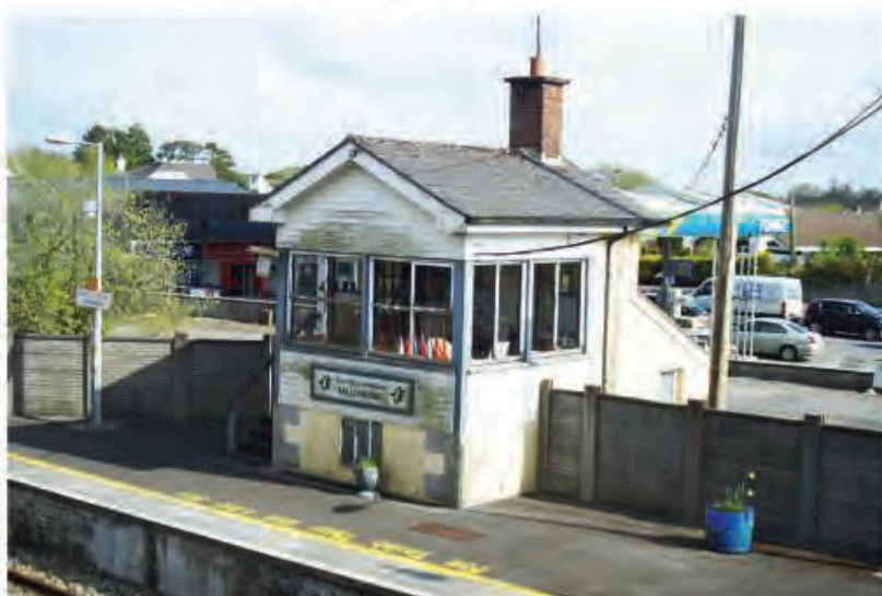
The signal box.
