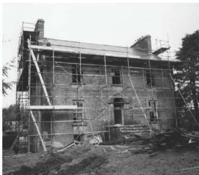
Taken during renovations.
