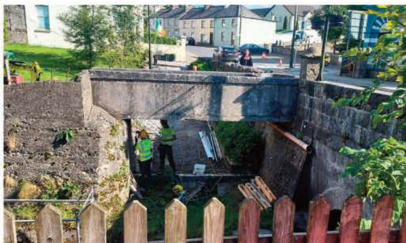
Survey work being undertaken at the old footbridge accessing the Friary Grounds from Bridge Street, with a view to its refurbishment, July 2024.
