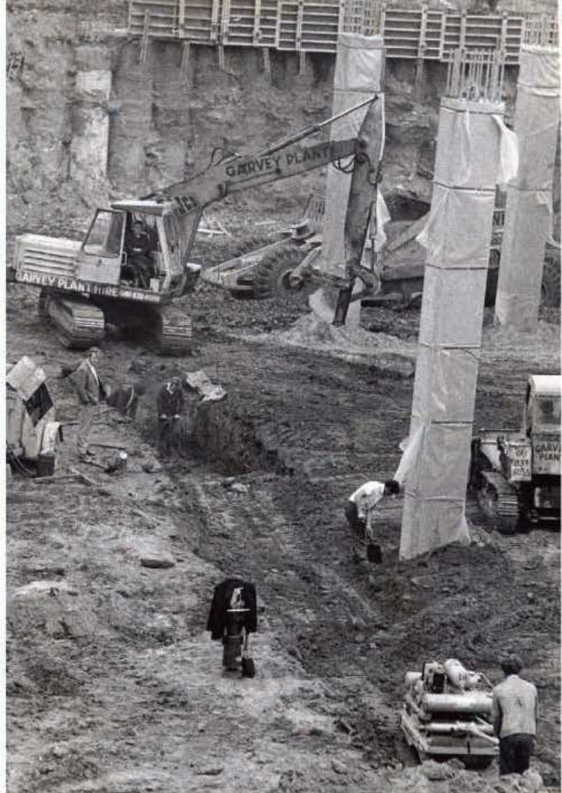
Oliver driving a track machine for Garvey's Construction on the Kingsway Bypass, 1960s.
